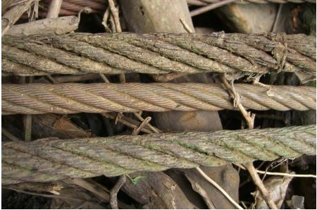
Figure 9: Cables from Old Bridge
