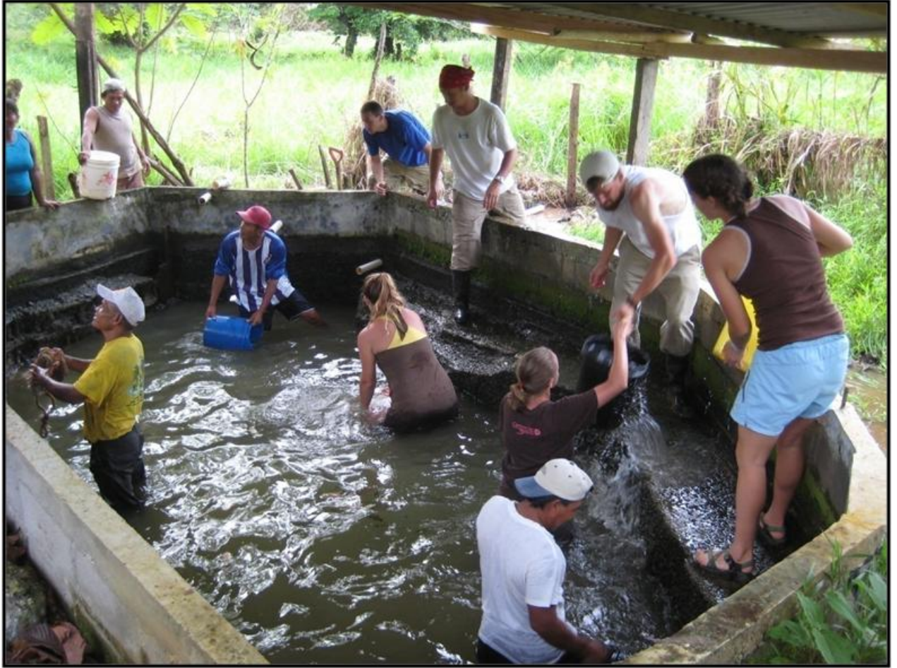
Image 3: Emptying and cleaning of existing toma . Photo by Ashley Thode.
