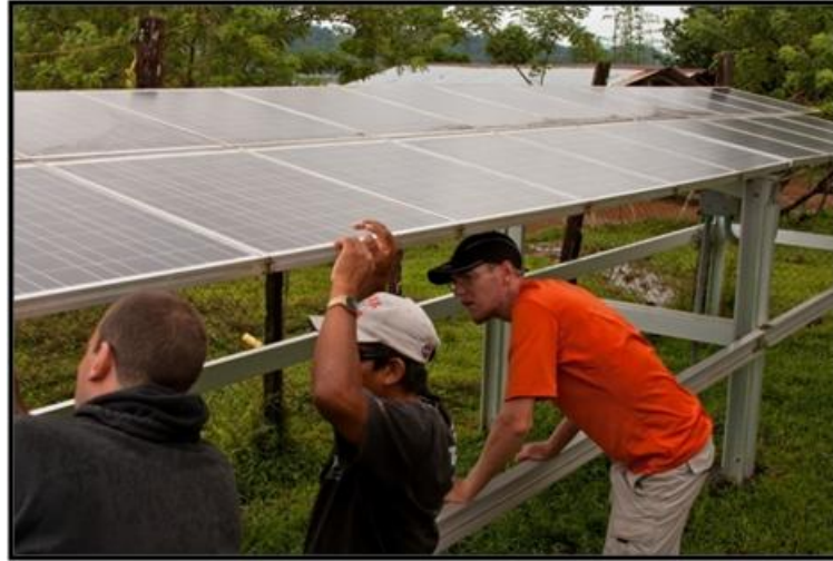
Image 7: Doctor’s office PV system 1. Photo by Kristian Bartell.
