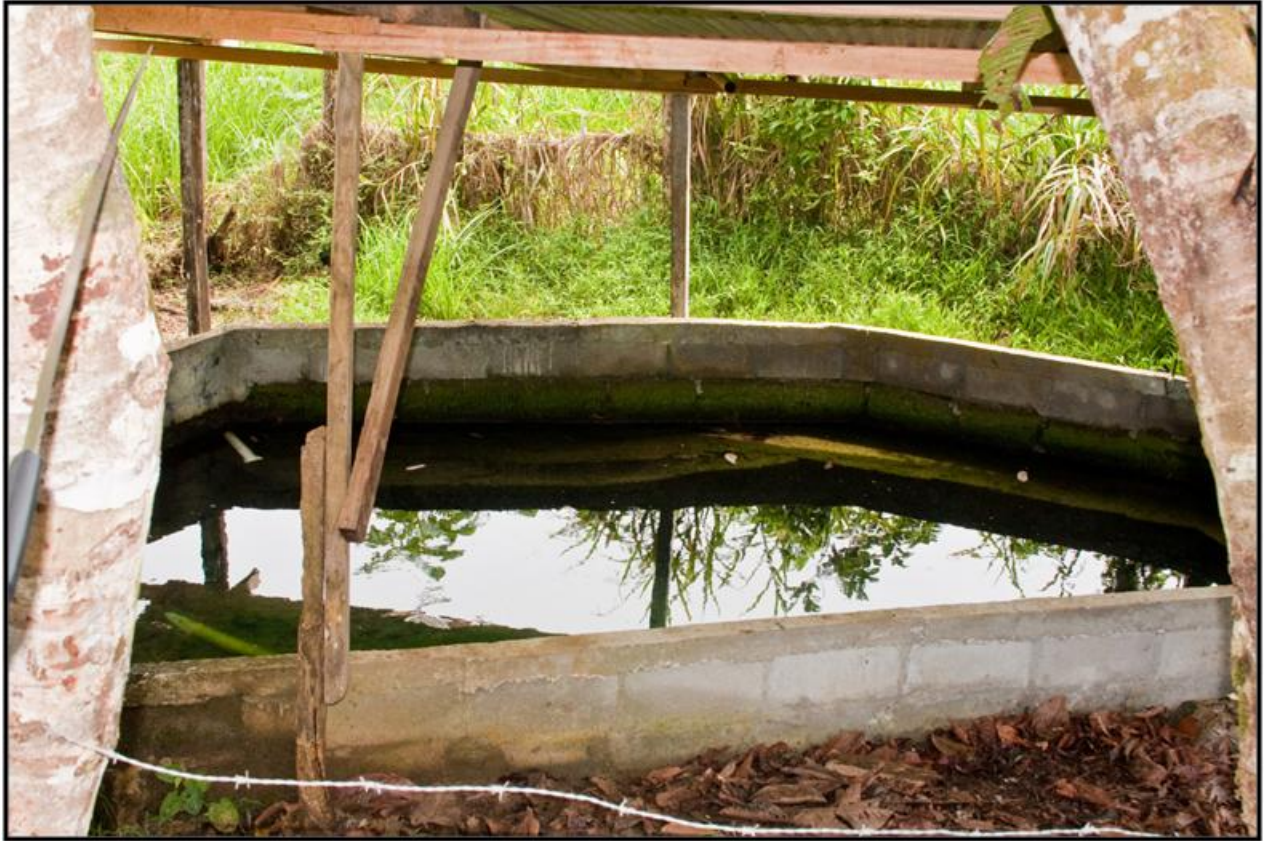
Image 1: Existing toma with a volume of 6,000 gallons (23,000 liters). Photo by Kristian Bartell.
