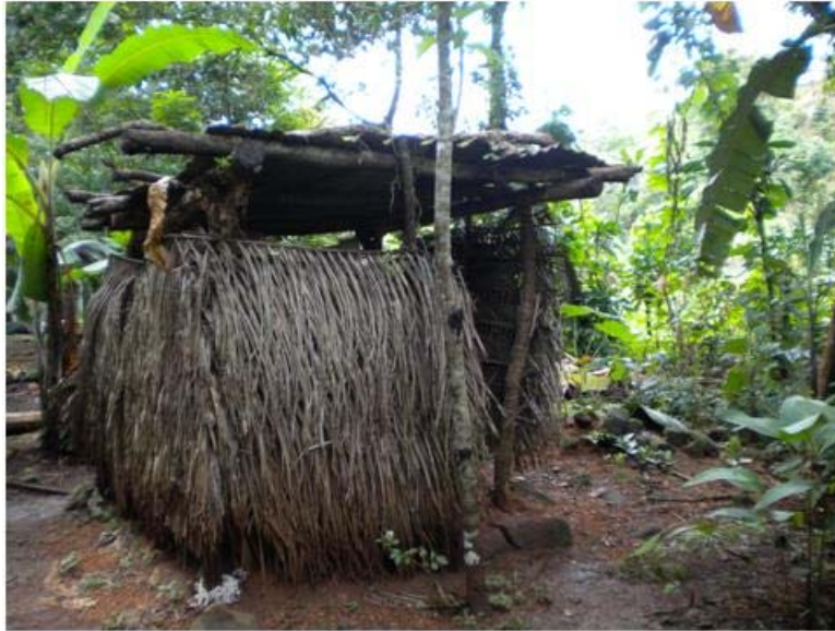
Figure 8: Example pit latrine built in Calabazal.
