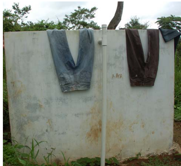
Figure 9: Quebrada Miña's water storage tank.
