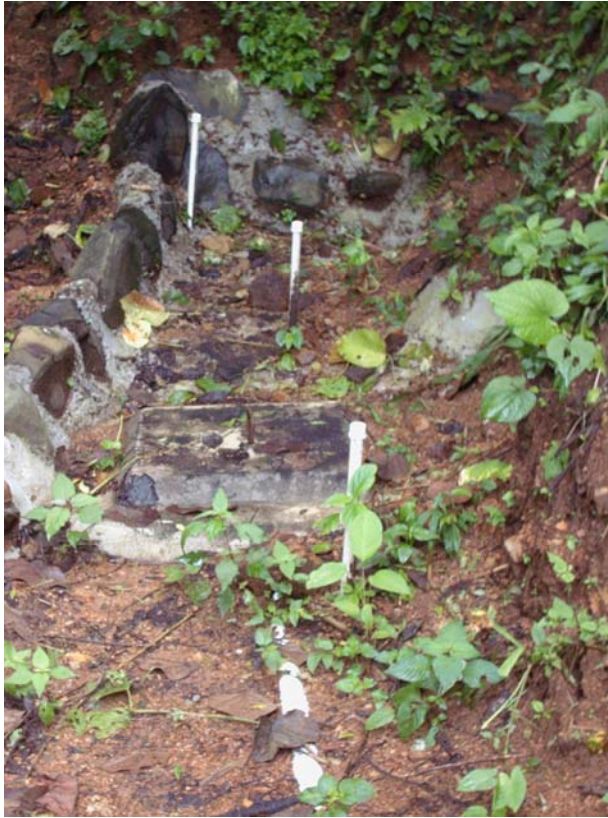
Figure 12: One of Quebrada Mina's Spring Boxes
