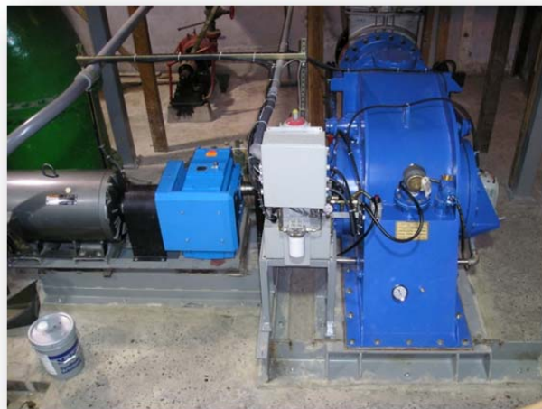
Figure 12: Canyon Hydro Cross Flow Turbine Picture Taken by Eric Melander [8],
