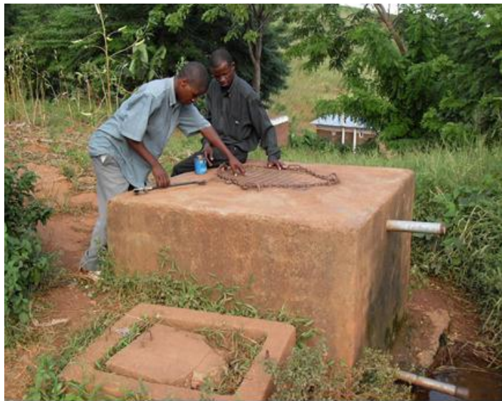
Figure 10: Example of Mason-Break Pressure Tank [Barefooteconomics.com]
