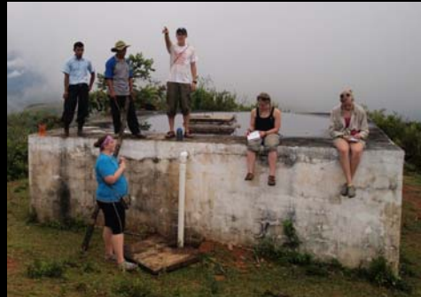
Storage tank for the new system in Cerro Miel Photo by Merete Sørum
