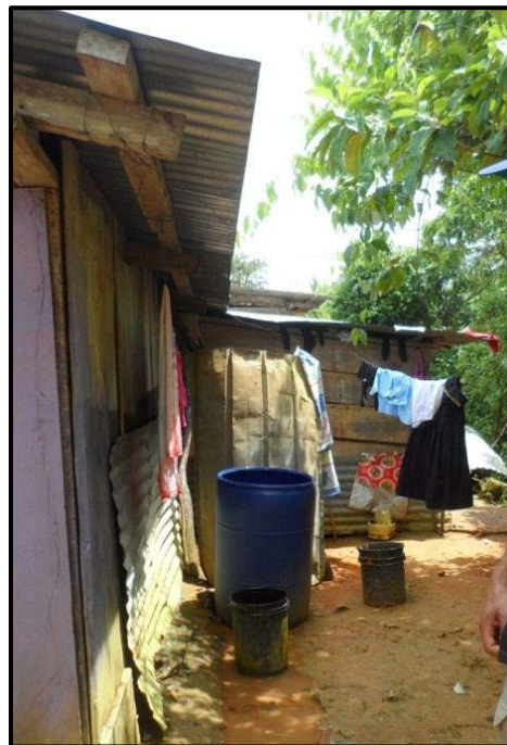
Figure 7 Example of rain water collection noted by the team at the store in Hato Pilón
