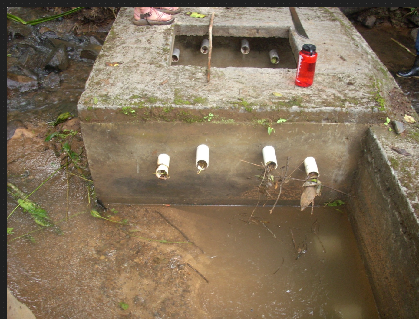
Existing small Intake structure attached to dam.
