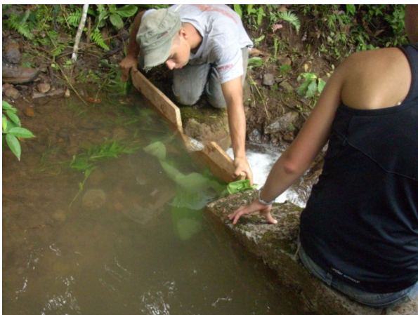
Figure 8. Weir on Spillway of Dam
