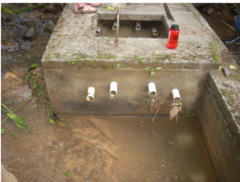
Figure 3. Current intake structure attached to the dam.
