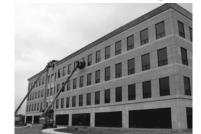
This is how the building will look after it is completed. The structural steel frame is one of the most important parts of the building. Building with steel has several advantages over other building materials. Steel can be erected year round. It is light yet strong when compared with other structural frame materials. Steel can also be adapted to almost any imaginable shape. One of the biggest advantages is that it can be erected very fast.
