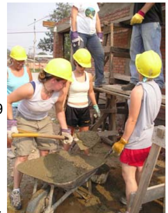
International Senior Design students building a classroom in Bolivia
