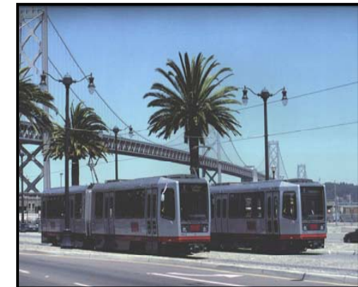
San Francisco MUNI Light Rail System
