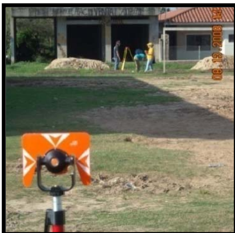
Figure 5: Surveying the Site
