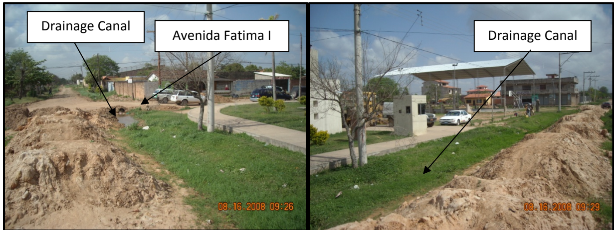
Figure 30: Existing Drainage Canal
