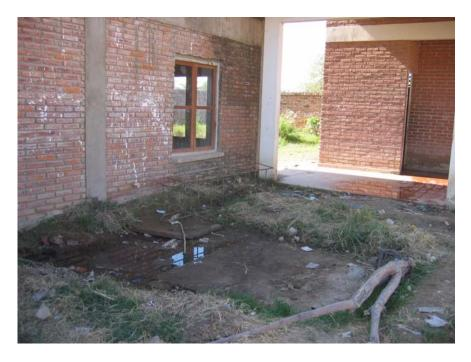
Figure 3: Existing septic tank with standing water
