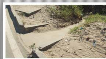
3. Existing curb inlet design
