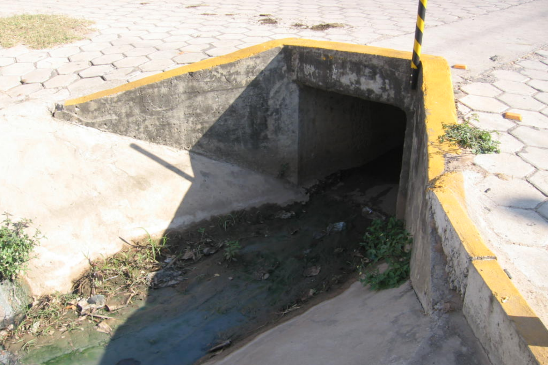
CONCRETE CANAL ALONG SAN MARTIN
